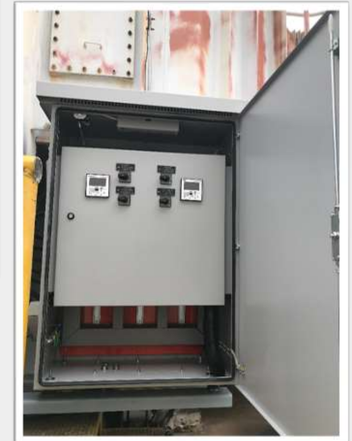
Temperature Monitor and Voltage Regulator Installation
